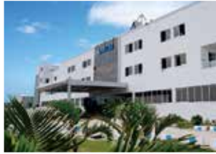
Rudrapur Plant (Green Building)
